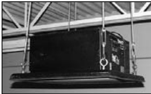
Figure 14: Levelled subwoofer
